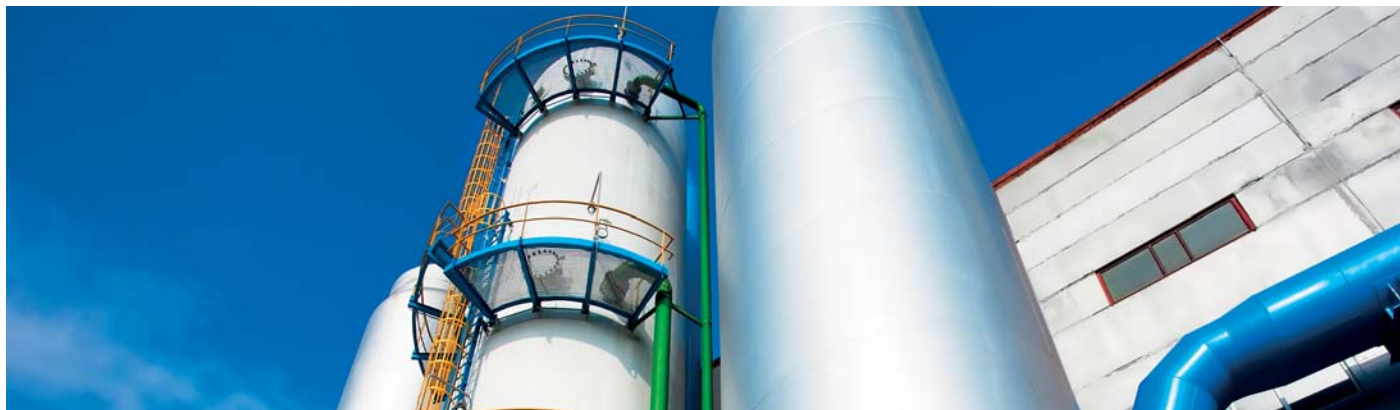
Air Separation Plant
